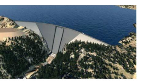
could be raised with a vertical extension of the upstream face, then a flattening of the downstream face to 0.70:1 for the second phase, 12m raise, and finally to 0.73:1 as part of the third phase for an additional 24m raise. This approach had the distinct advantage of permitting future raised construction without significantly lowering the reservoir, which would be needed for water supplies during the construction period.
